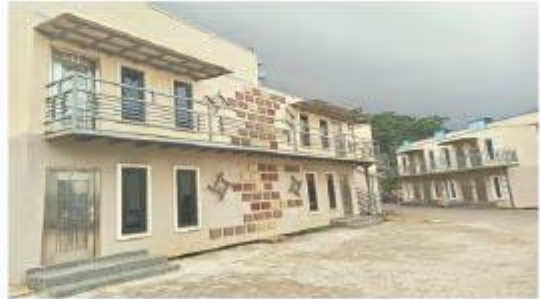
Newly installed Portacabins
