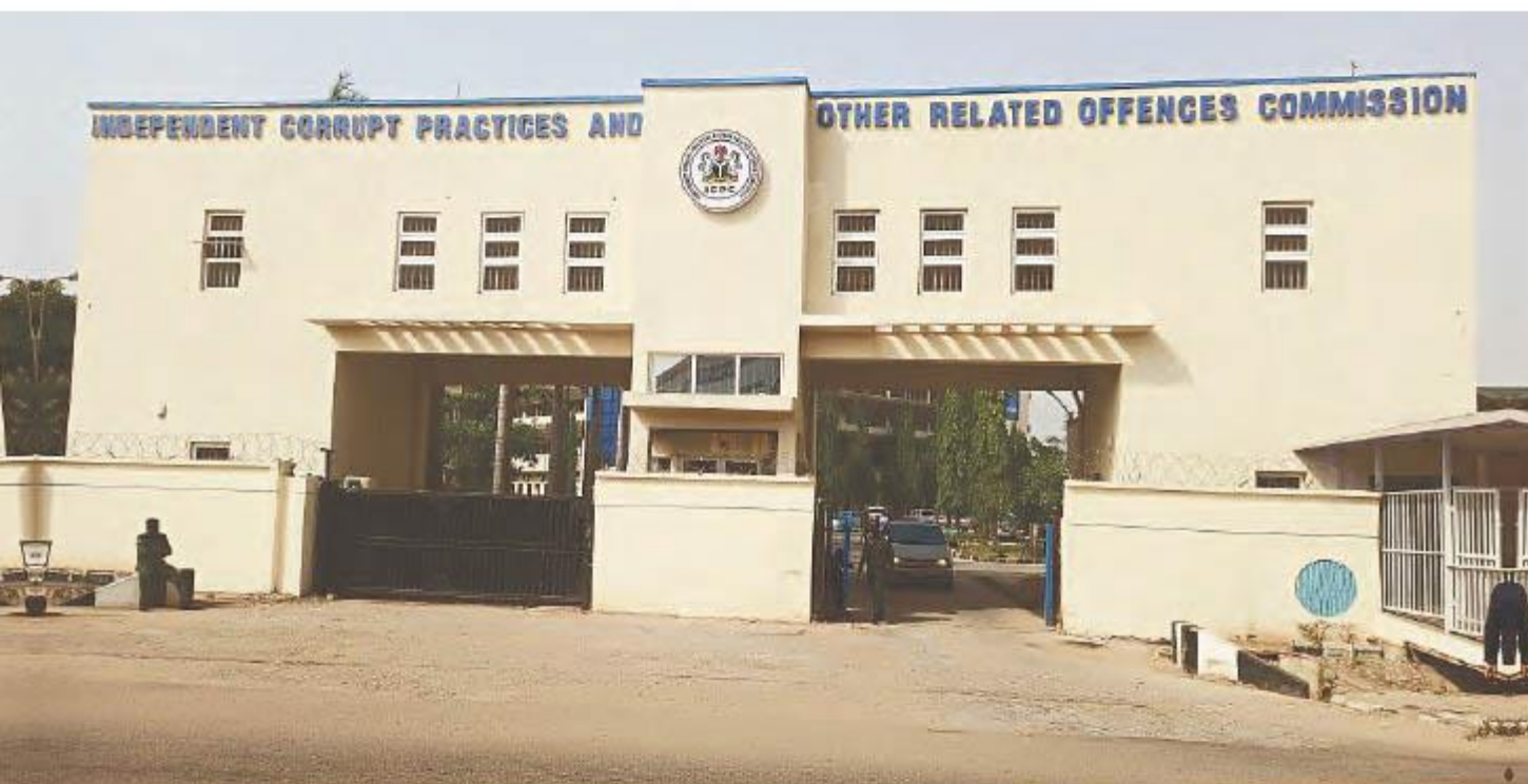
Newly Constructed Gatehouse
