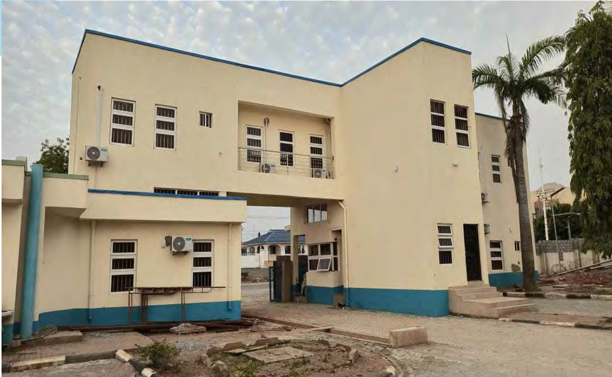
New Main Gate
